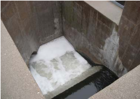
Water leaving treatment plant
